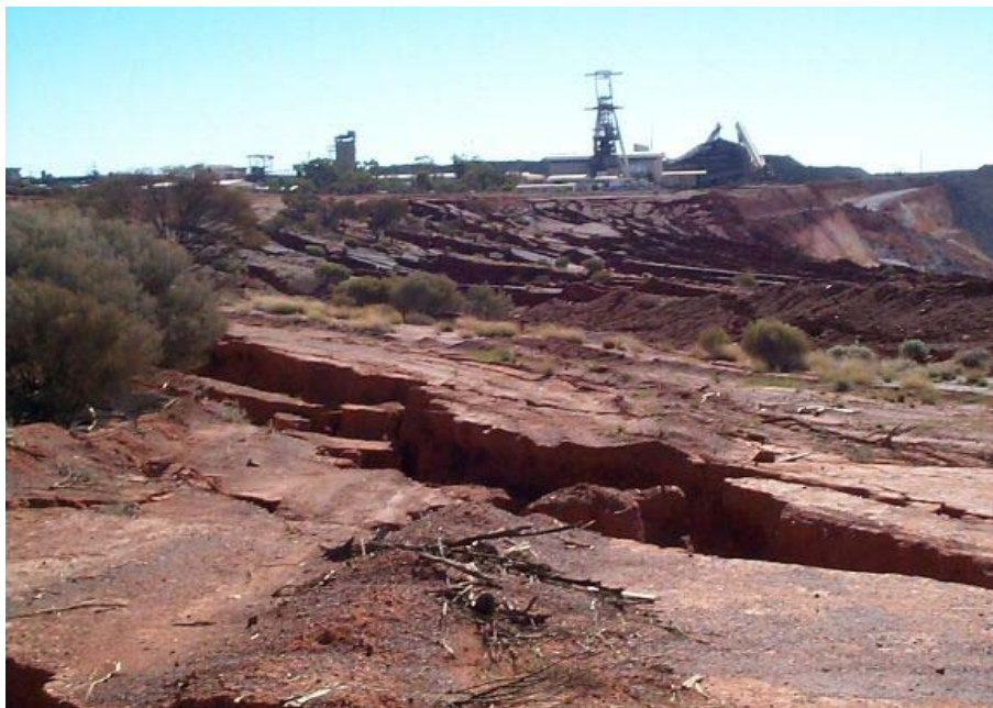
Figure 7: Large surface deformations next to an open pit mine.
