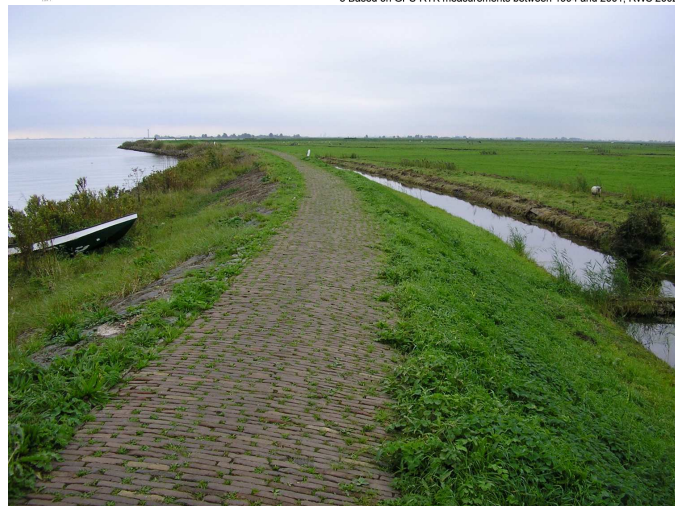
Fig. 2. Top: Leveling, GPS, and PSI measurements over the dike protecting the former island of Marken. Bottom: photograph of the physical appearance of the dike.
