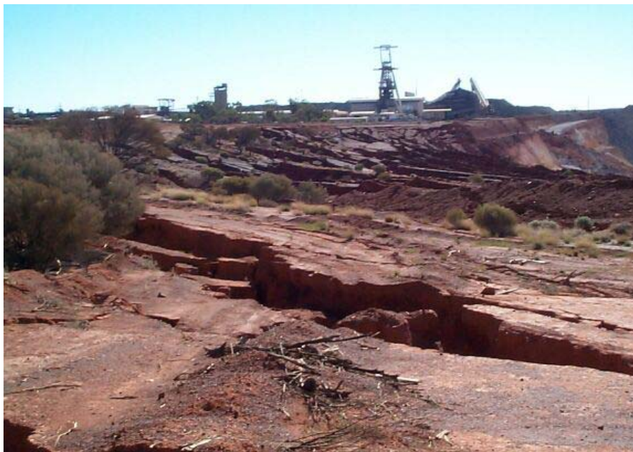
Figure 1: Large surface deformations next to an open pit mine.
