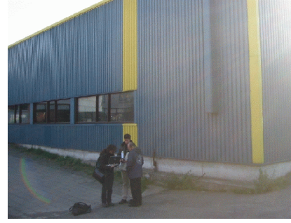
Figure 7: Field test to validate a local subsidence: here it is the premise that is subsiding instead of the building.
