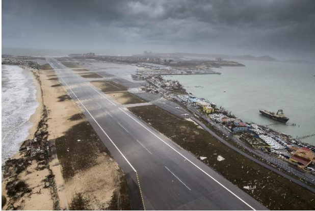
Figure 22: Beach at Simpson Bay where most of the sand has shifted on the landing strip (NRC, 2017)
