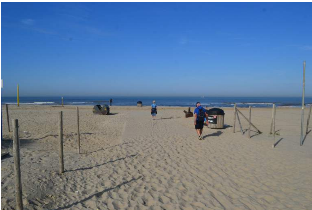
Figure 41: This photograph shows that there can also be a lot of sand covering the concrete slabs located around the beach entrances. Photograph was taken at Kijkduin beach on the 16th of October.
