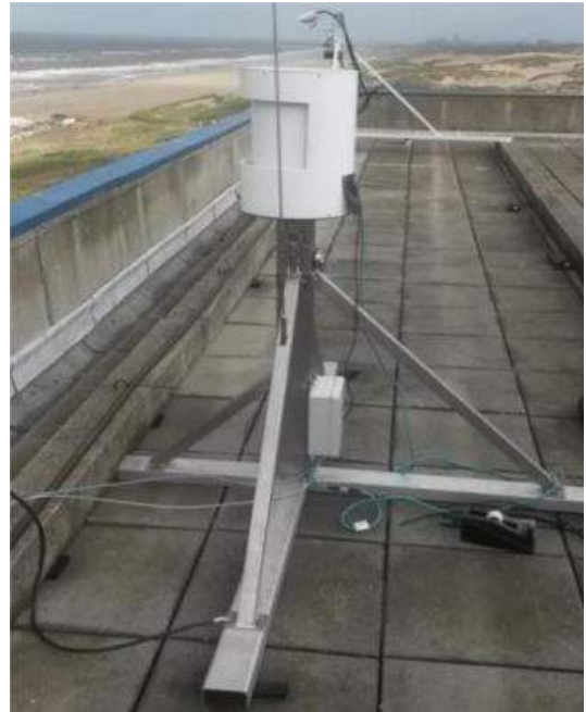
Figure 6: The Riegl-VZ 2000 laser scanner on top of Hotel NH Atlantic Den Haag at the test location (after (Vos et al. 2017))
