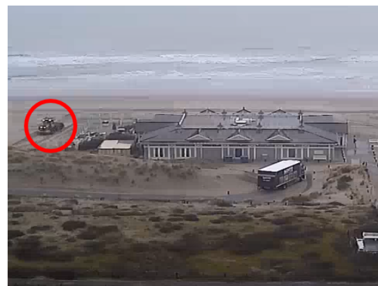
(b) A bulldozer is present in the area of deformation.
