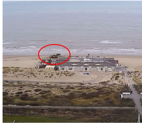
(b) A bulldozer is present in the area of deformation.
