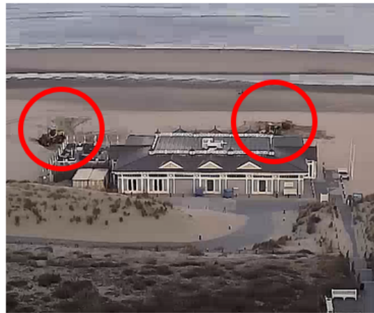
(b) Two bulldozers are present and working in the area of deformation.
