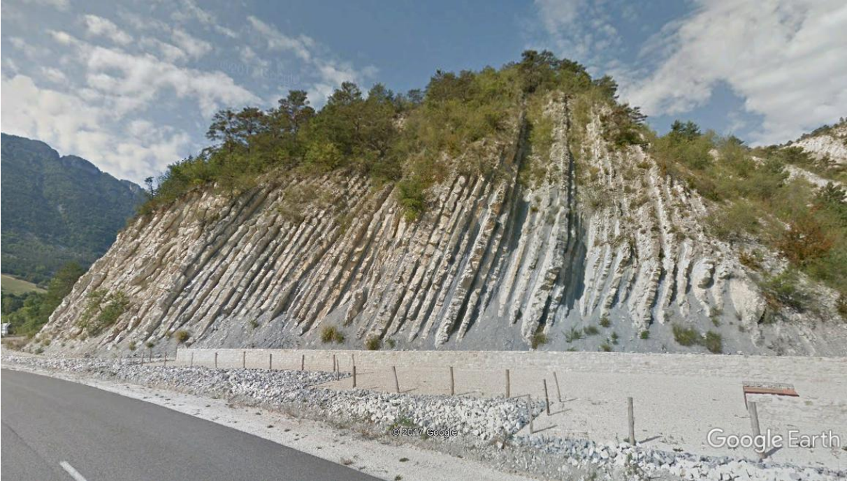
Figure 4: Google street view image of the outcrop
