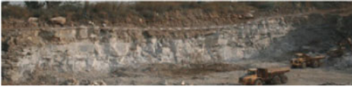
Figure 1. East face of the Dan quarry after the blast. The face is about 10 m high. It is intersected by at three dominant discontinuity sets, two subvertical and one subhorizontal sets with a mean true spacing of 4.3, 0.5 and 1 m, respectively and a less dominant diagonal set.
